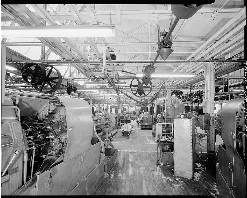
Photo: Machine shop with original line shafting and belts, White Company, Cleveland. Library of Congress, HAER OHIO,18-CLEV,25C-24 — no known restrictions
